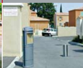
Access control unit
